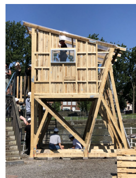
⑤ Assembling: the sauna takes shape within five days.
